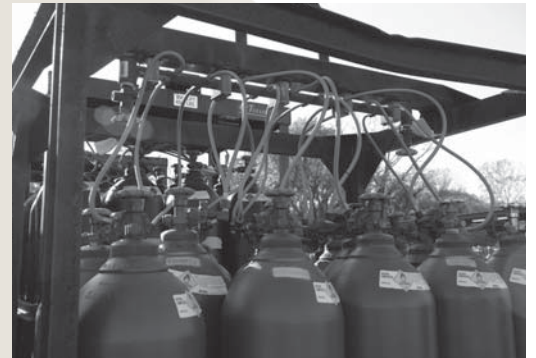
HIGH PRESSURE OXYGEN BANK
