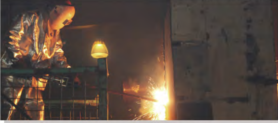
Demolition of Injection Mold Machine 450 tons of steel ranging from 4 to 26 inch thick.
